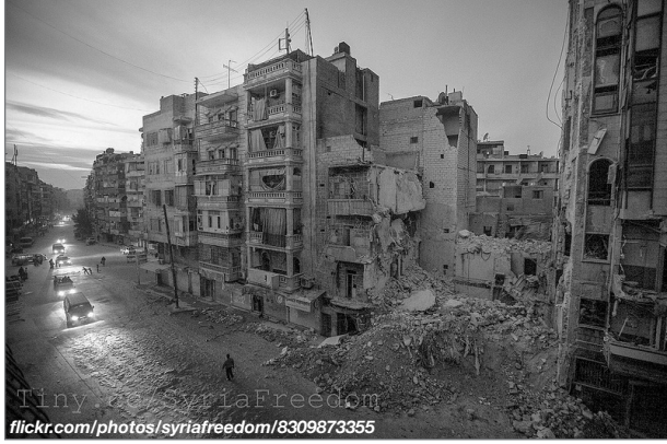
Dar Al-Shifa hospital, Syria, (at the right of the frame) has been bombed and shelled more than 20 times. It is now a symbol of resistance.
