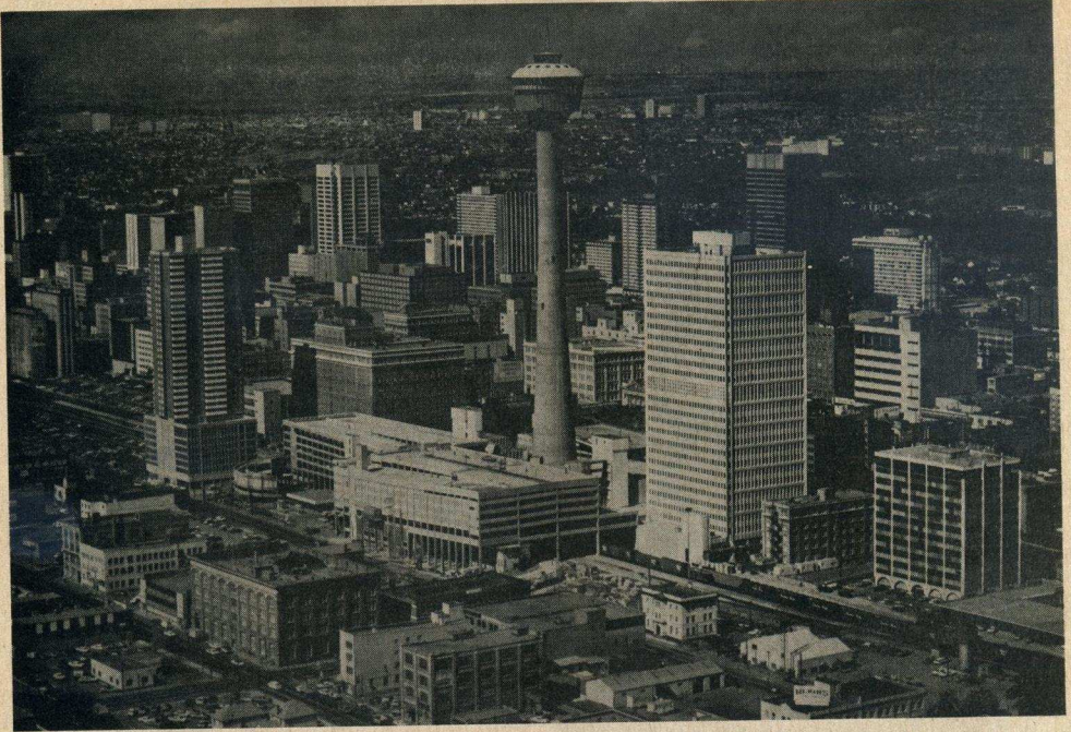
This view of downtown Calgary is dominated by Canadian Pacific buildings. The Husky Tower (owned by Canadian Pacific despite its name) and Palliser Square are in the centre.
